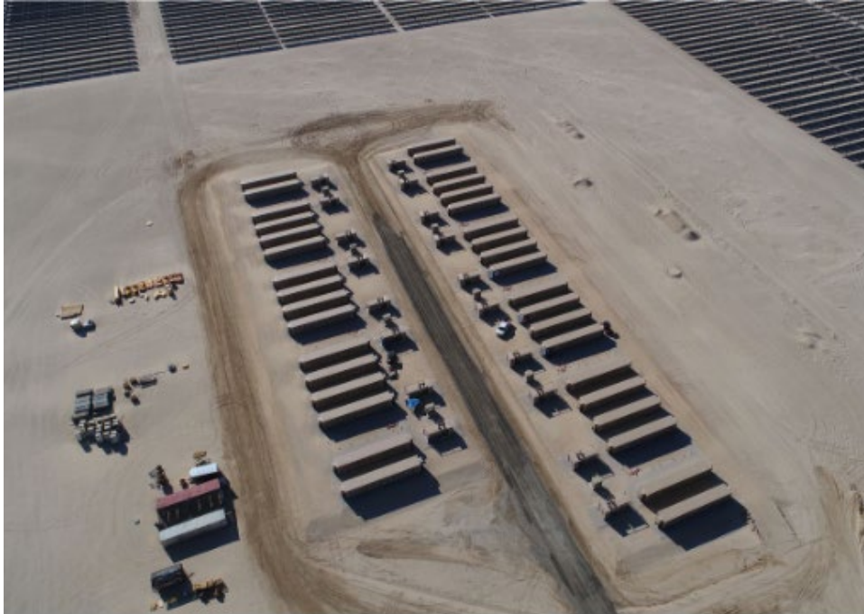
Figure 1. Maverick Solar 6 Battery Storage Component Under Construction
